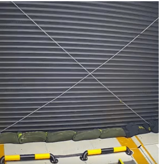
NIO Power Swap Station With Temporary Reinforcement Against Typhoons
